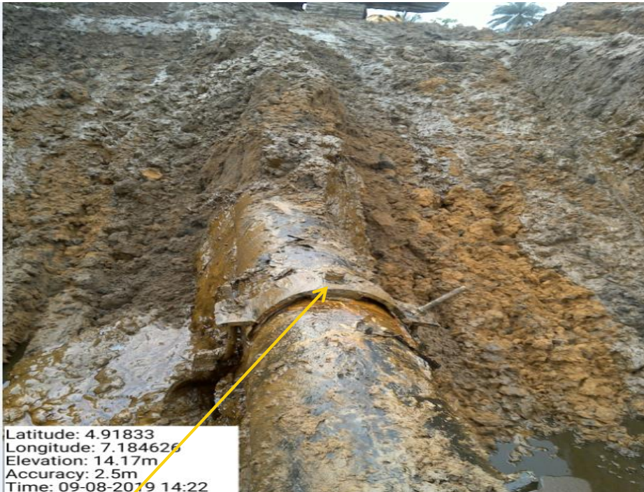
Close-up: Illegal fitting on 12'' Imo River - Ogale Pipeline at Okohia. Picture was taken during Joint Investigation of 8 th September 2019
