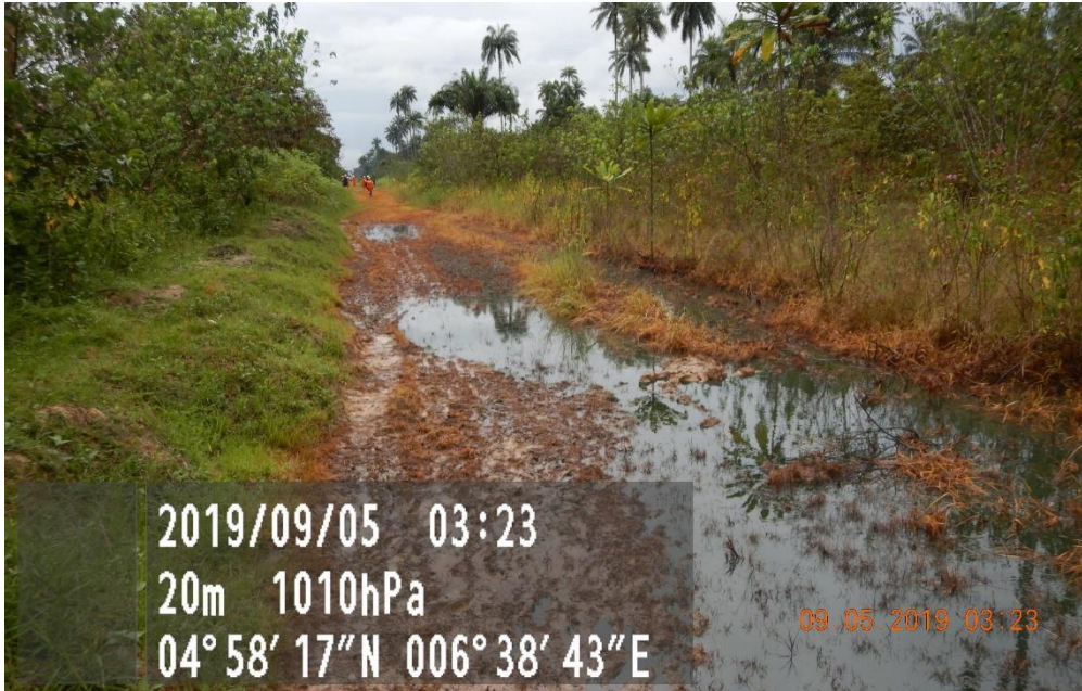
Overview: Part of spill impact on New 20" Kolocreek - Rumuekpe Pipeline Right of Way at Okoma1 . Picture was taken during Joint Investigation of 5 th September 2019.
