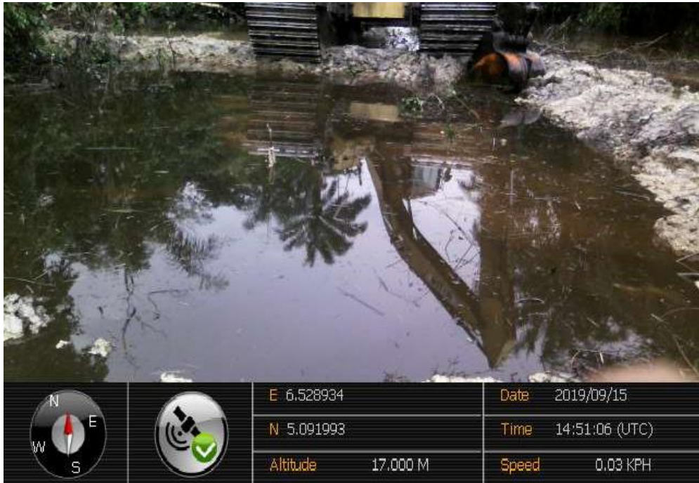
Overview: Part of spill impact on 14" Okordia - Rumuekpe Pipeline Right of Way at Ukpeliède. Picture was taken during Joint Investigation of 15 th September 2019.
