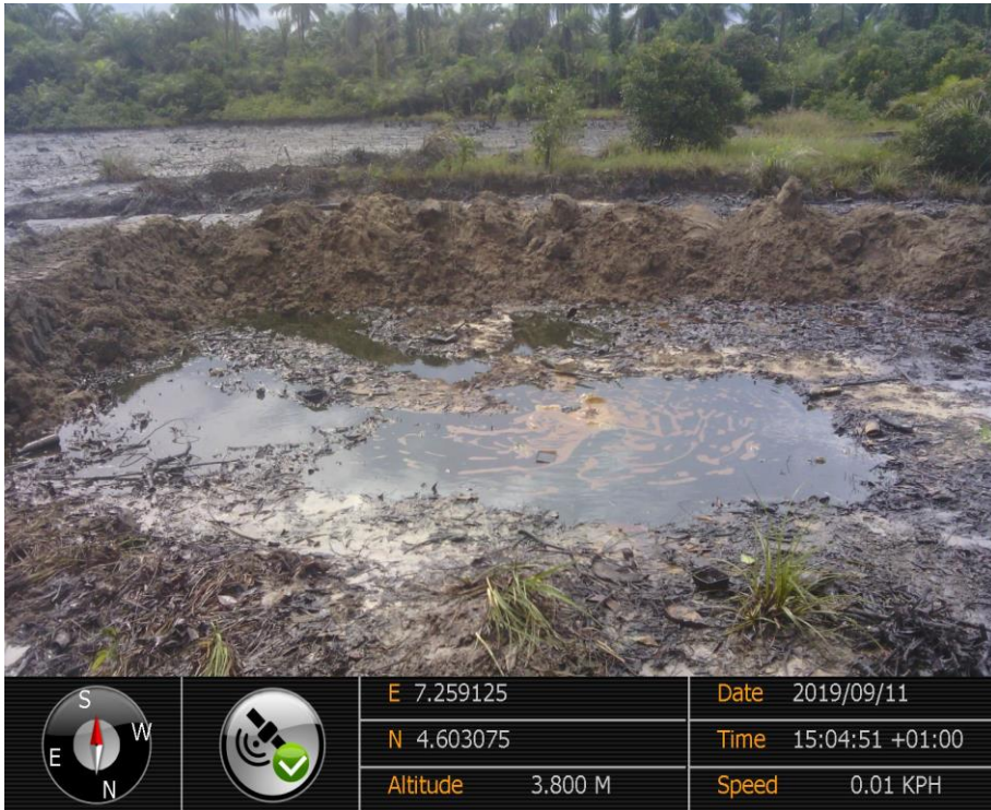
Overview: Part of spill impact on 24" Bomu - Bonny Pipeline Right of Way at Patrick Waterside_Bodo West. Picture was taken during Joint Investigation of 11 th September 2019.
