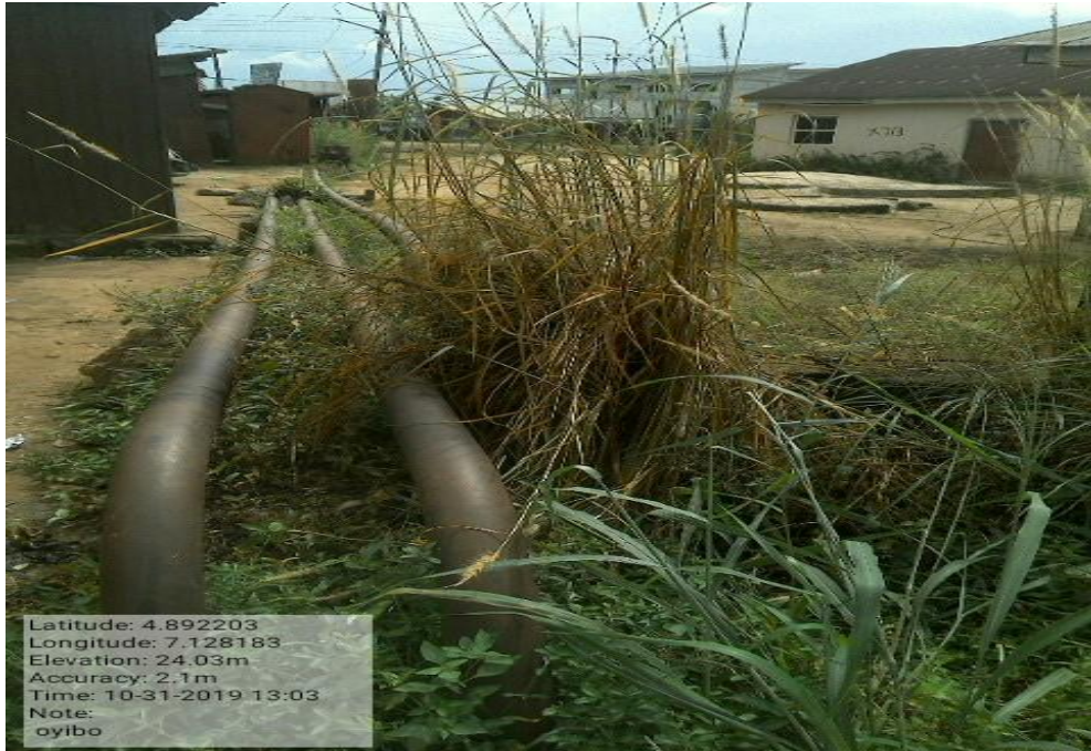
Overview: Part of spill impact on 4" Obigbo Well 38 & 52 Flowline at Umuebulu. Picture was taken during Joint Investigation of 31 st October 2019.
