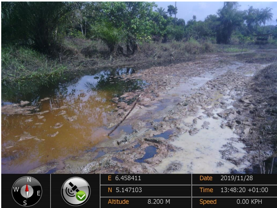
Overview: Part of spill impact on 14inch Okordia Rumuekpe Pipeline at Ikarama. Picture was taken during Joint Investigation of 28 th November 2019.
