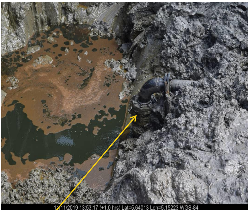
Close-up: Illegal Fitting on 20 " Trans – Escravos at Ugboegungun. Picture was taken during Joint Investigation of 11 th November 2019
