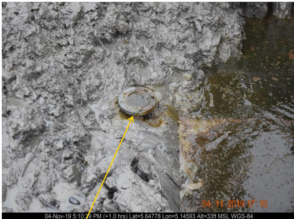
Close-up: Illegal Fitting on 20'' Trans - Escravos Pipeline at Ugboegungun. Picture was taken during Joint Investigation of 4 th November 2019.
