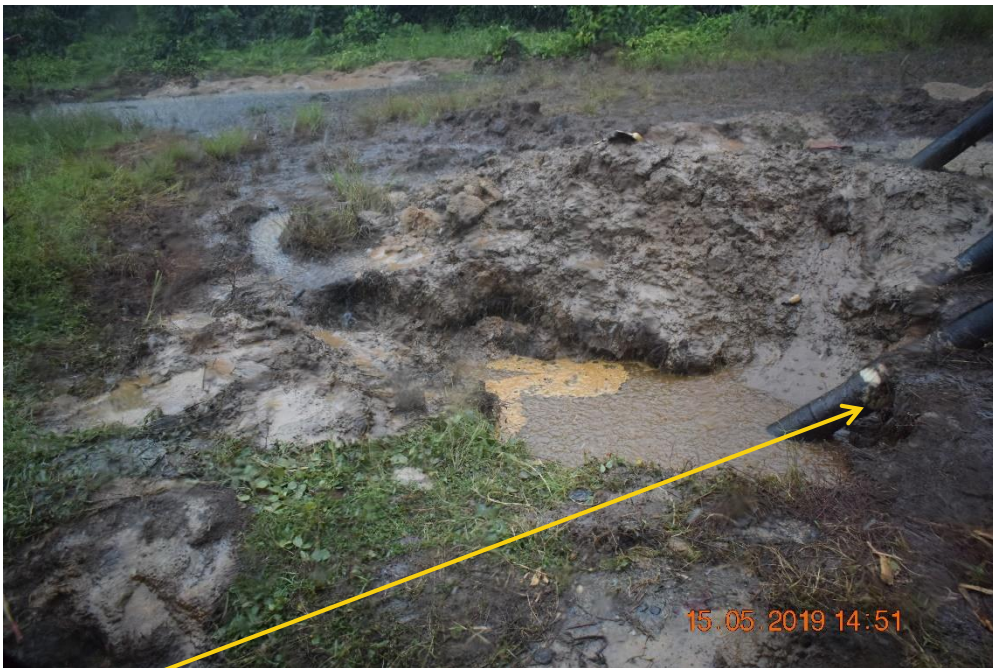
Close-up: Corrosion on Yokri LP1 bulk-line manifold 8 at Yokiri. Picture was taken during Joint Investigation of 15 th May 2019
