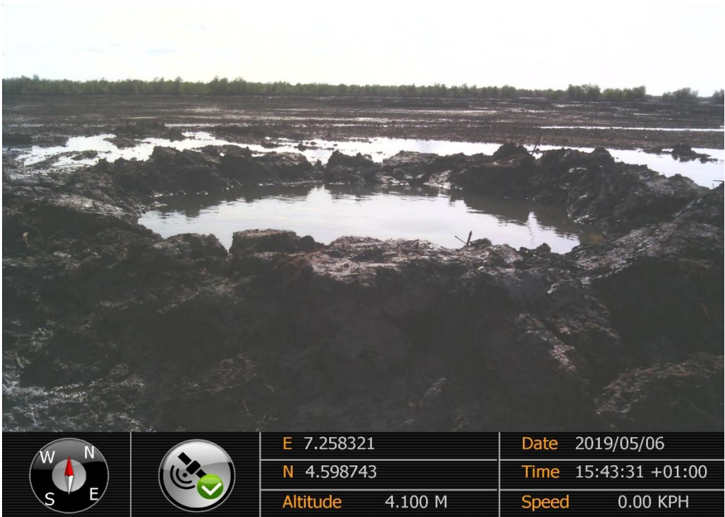
Overview: Part of spill impact on 24" Bomu – Bonny Pipeline Right of Way at Patrick Waterside - Bodo West. Picture was taken during Joint Investigation of 6 th March 2019.
