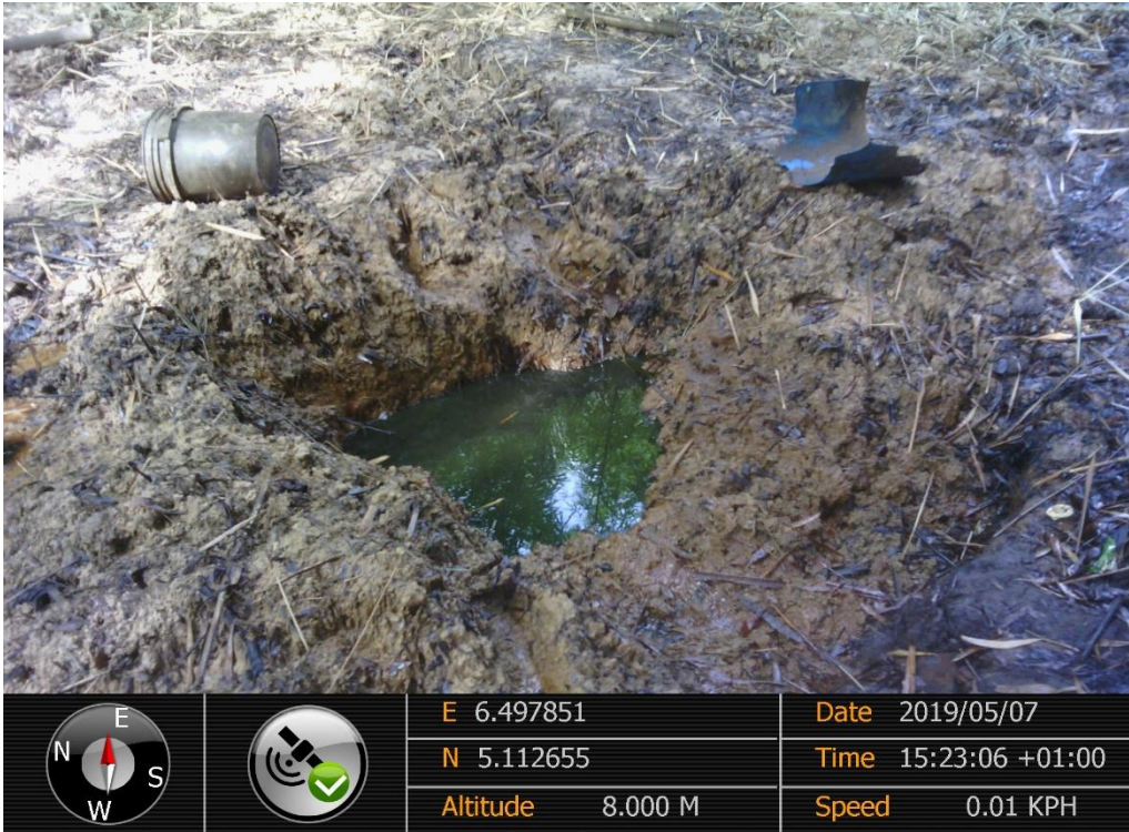
Overview: Part of spill impact on 14" Okordia - Rumuekpe Pipeline Right of Way at Akala-Olu. Picture was taken during Joint Investigation of 7 th May 2019.
