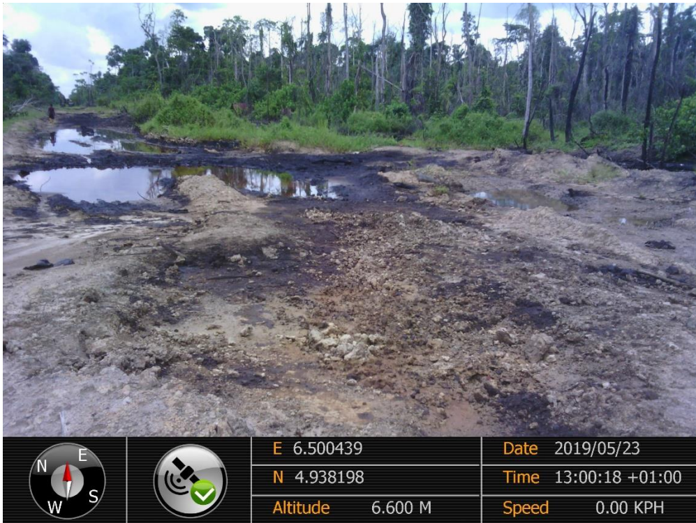
Overview: Part of spill impact on 20'' Kolocreek – Rumuekpe Pipeline Right of Way at Odau. Picture was taken during Joint Investigation of 23 rd May 2019
