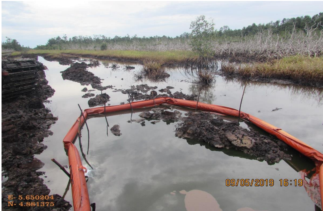
Overview: Part of spill impact on 6'' Tunu Kanbo Well 7L Flowline at Egbemo-Analabiri-agbidiana. Picture was taken during Joint Investigation of 9 th May 2019.
