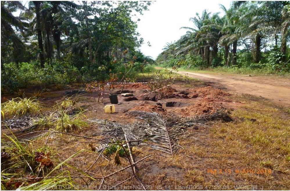
Overview: Part of spill impact on 16" Egbema - Assa Pipeline Right of Way at Obile. Picture was taken during Joint Investigation of 9 th April 2019.
