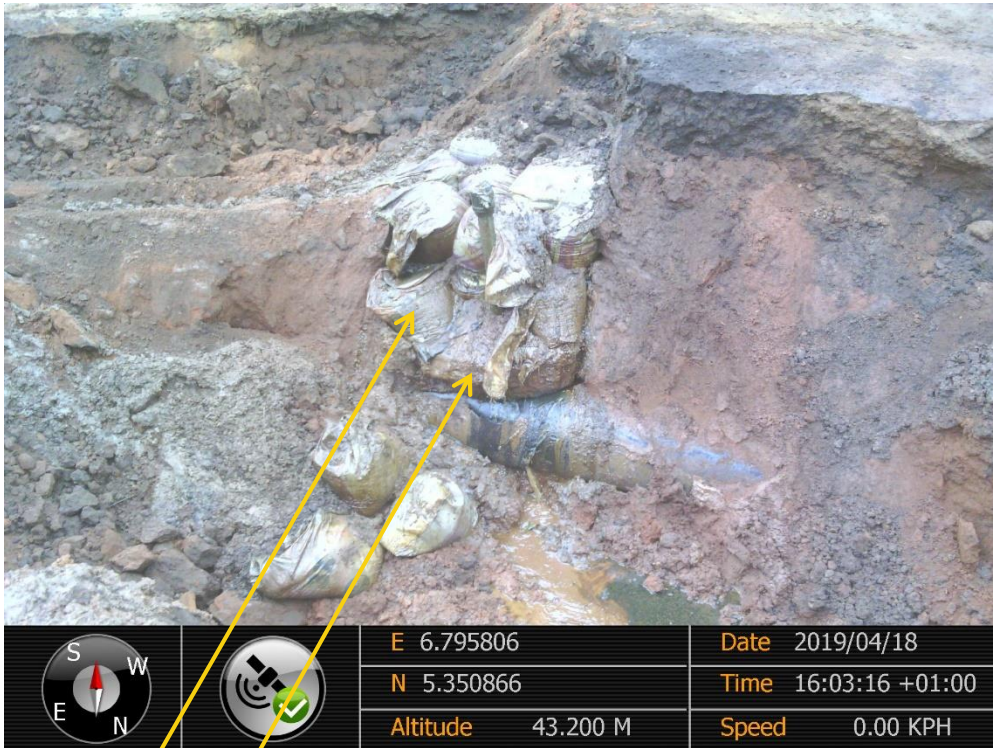
Close-up: Sand bag and Concrete concealing theft point on 18" Assa – Rumuekpe Pipeline at Ochia-Awarra. Picture was taken during Joint Investigation of 18 th April 2019
