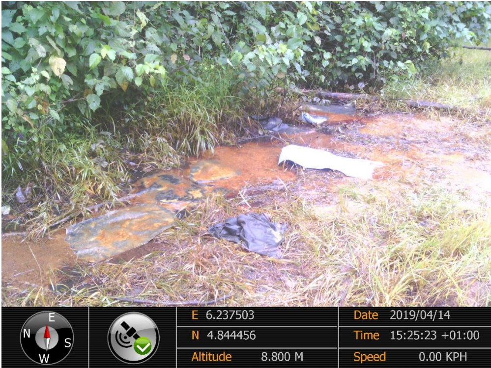
Overview: Part of spill impact on 16" Nun River - Kolocreek Pipeline Right of Way at Otuegwel. Picture was taken during Joint Investigation of 14 th April 2019.
