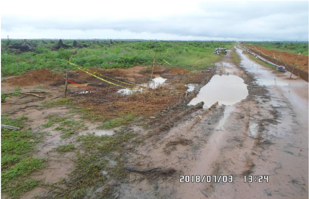
Overview: Part of spill impact on 18" Assa – Rumuekpe Pipeline Right of Way at Omudioga. . Picture was taken during Joint Investigation of 3 rd July 2018.
