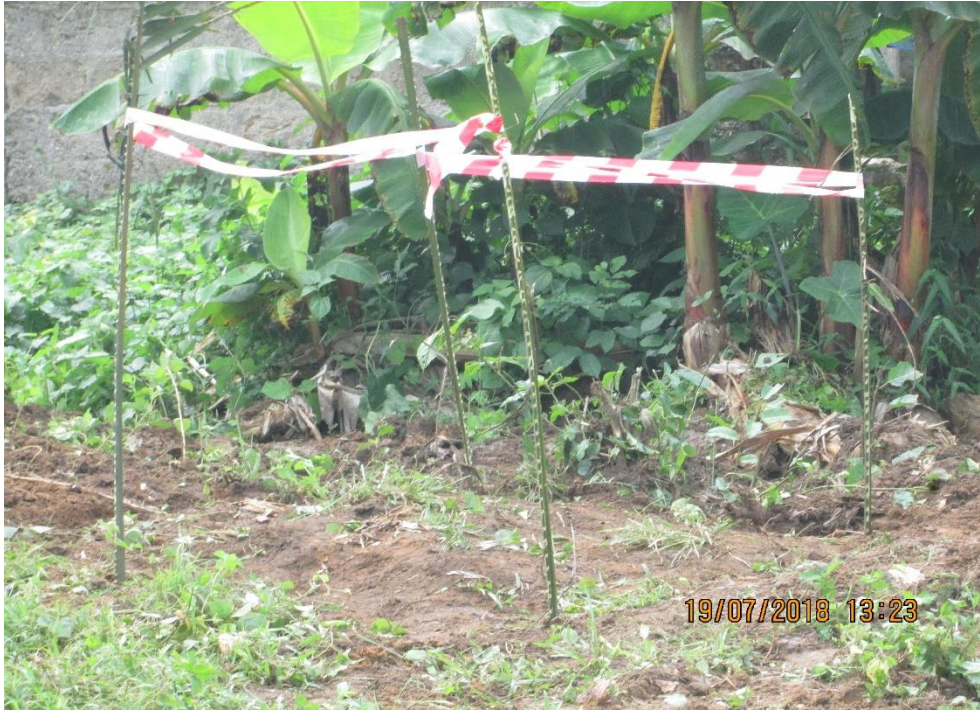
Overview: Part of spill impact on 20" Rumuekpe-Nkpoku Pipeline Right of Way at Mbodo-Aluu. Picture was taken during Joint Investigation of 19 th July 2018.
