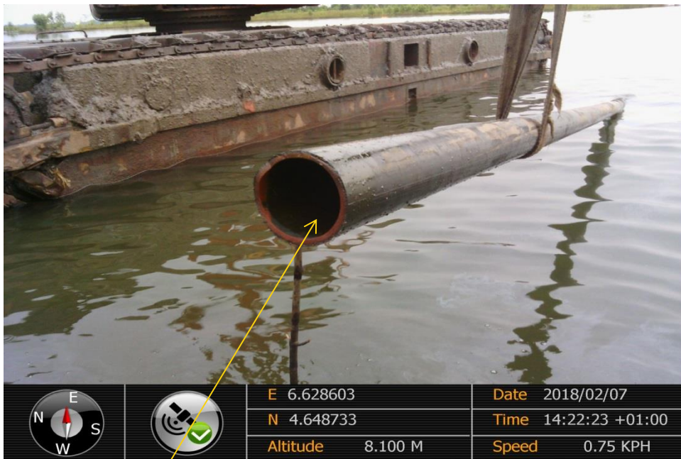
Close-up: Position of missing flowline on Soku Well 14S Flowline at Soku. Picture was taken during Joint Investigation of 7 th February 2018.
