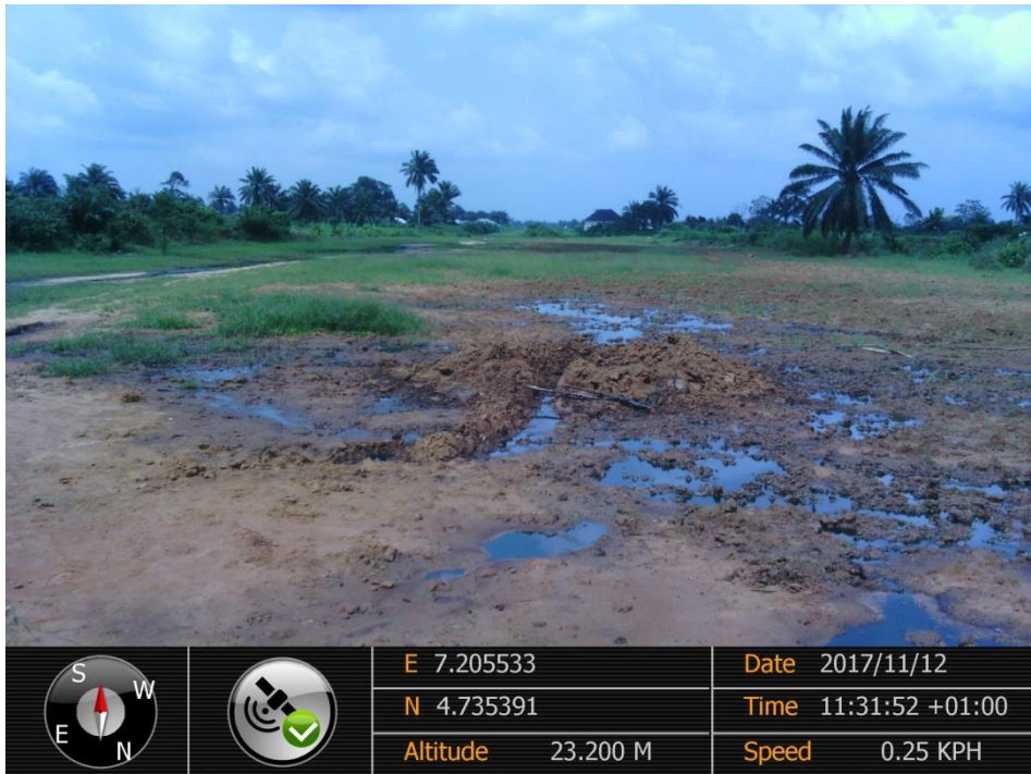
Overview: Part of spill impact on 28" Nkpoku-Bomu Pipeline Right of Way at Norkpo. Picture was taken during the Initial Site Visit of 12 th Nov. 2017.
