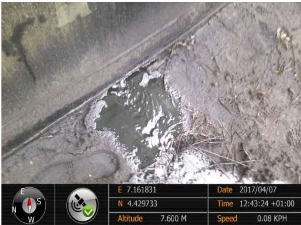
Close-up: Spill point within Bonny Oil & Gas Terminal Tank Bund area at Bonny. Picture was taken during Joint Investigation of 7 th April 2017.
