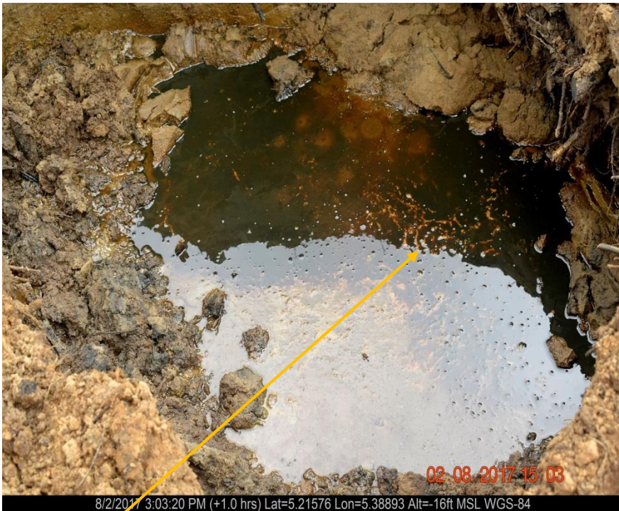
Close-up: Excavated Pit with residual oil seepage on 24"Trans-Ramos Pipeline at Odimodi. Picture was taken during Joint Investigation of 2 nd August 2017.
