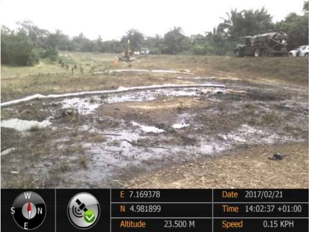
Overview: Part of spill impact on 12" Imo River2 – Ogale Pipeline Right of Way at Odagwa. Picture was taken during Joint Investigation of 21 st February 2017.
