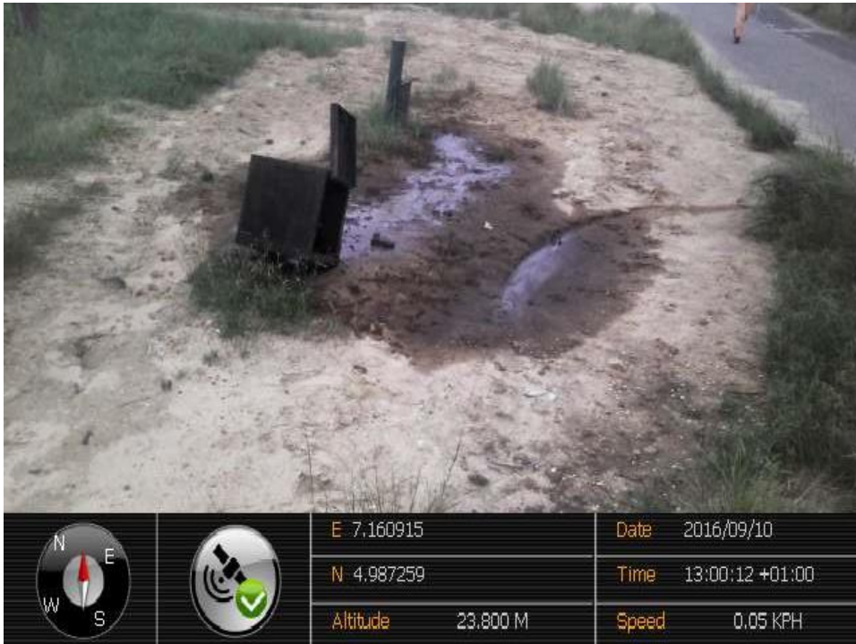
Overview: Part of spill impact on 8" Nkali-Imo River 2 Pipeline (Breathing Tube Box) at Umuedu-Okwara. Picture was taken during Joint Investigation of 10 th September 2016.
