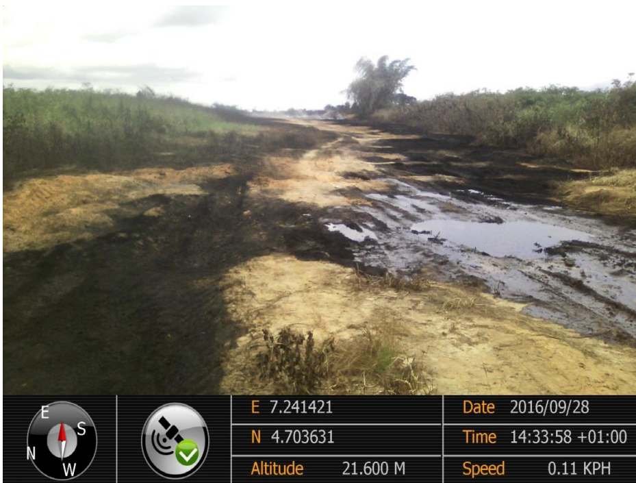
Overview: Part of spill impact on 28" Nkpoku-Bomu Pipeline at Gio. Picture was taken during Preliminary site visit of 28 th September 2016.
