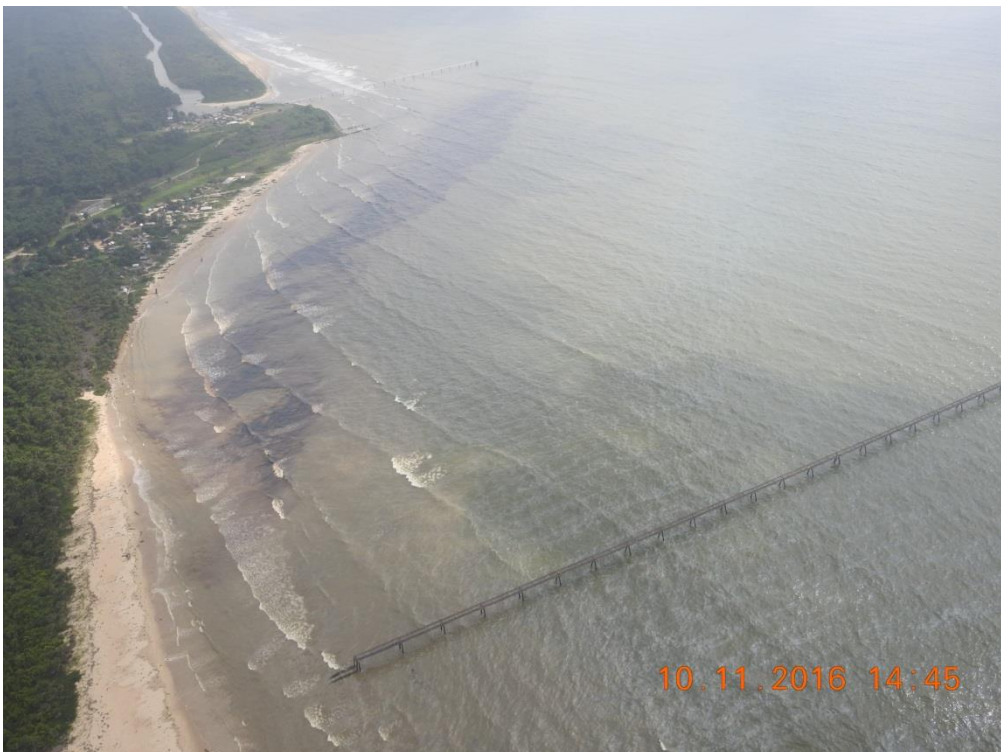
Overview: Part of spill impact on 48" Forcados Export Terminal Export Pipeline at Ogulagha. Picture was taken during overfly on 10 th November 2016.
