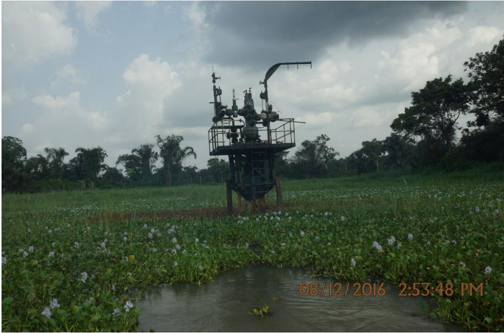
Overview: Part of spill impact on Benisede Well 6S Wellhead at Ojobo. Picture was taken during Joint Investigation of 8 th December 2016.
