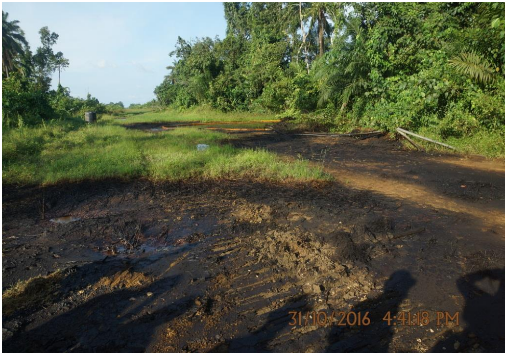
Overview: Part of spill impact on 20" Otumara-Escravos Pipeline at Ogidigben. Picture was taken during Joint Investigation of 31 st October 2016.
