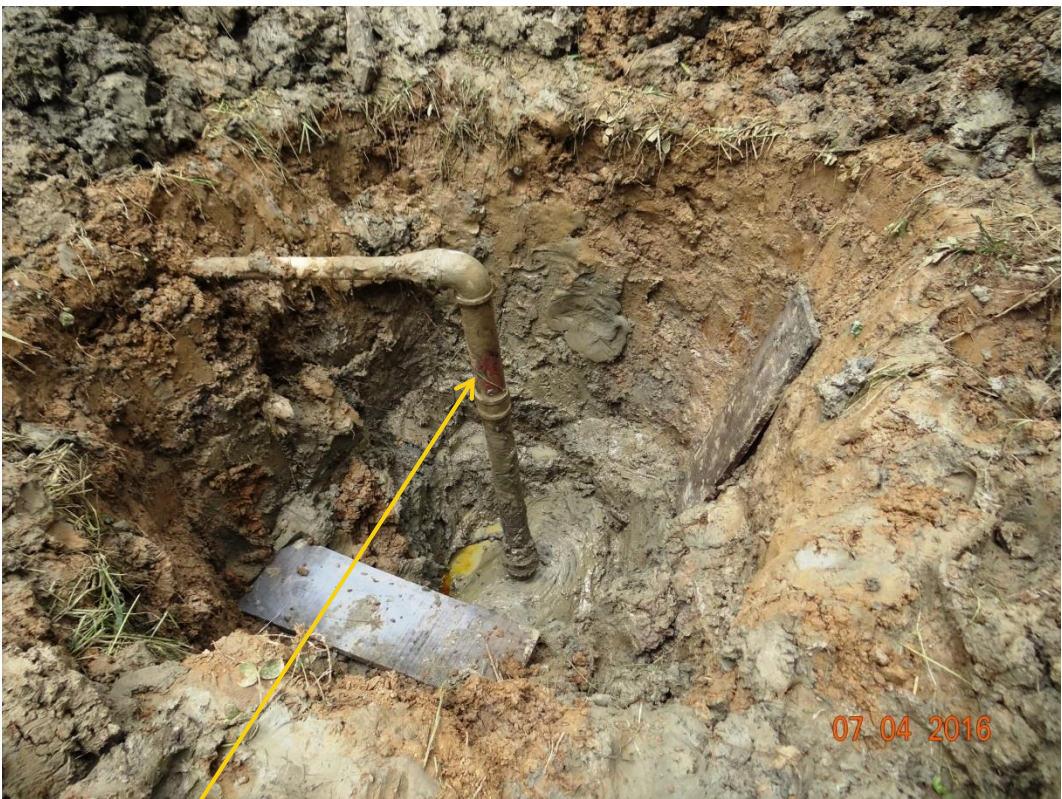
Close-up: Illegal fitting on 20" KoloCreek – Rumuekpe Trans Niger Pipeline at Odau. Picture was taken during Joint Investigation of 7 th April 2016.
