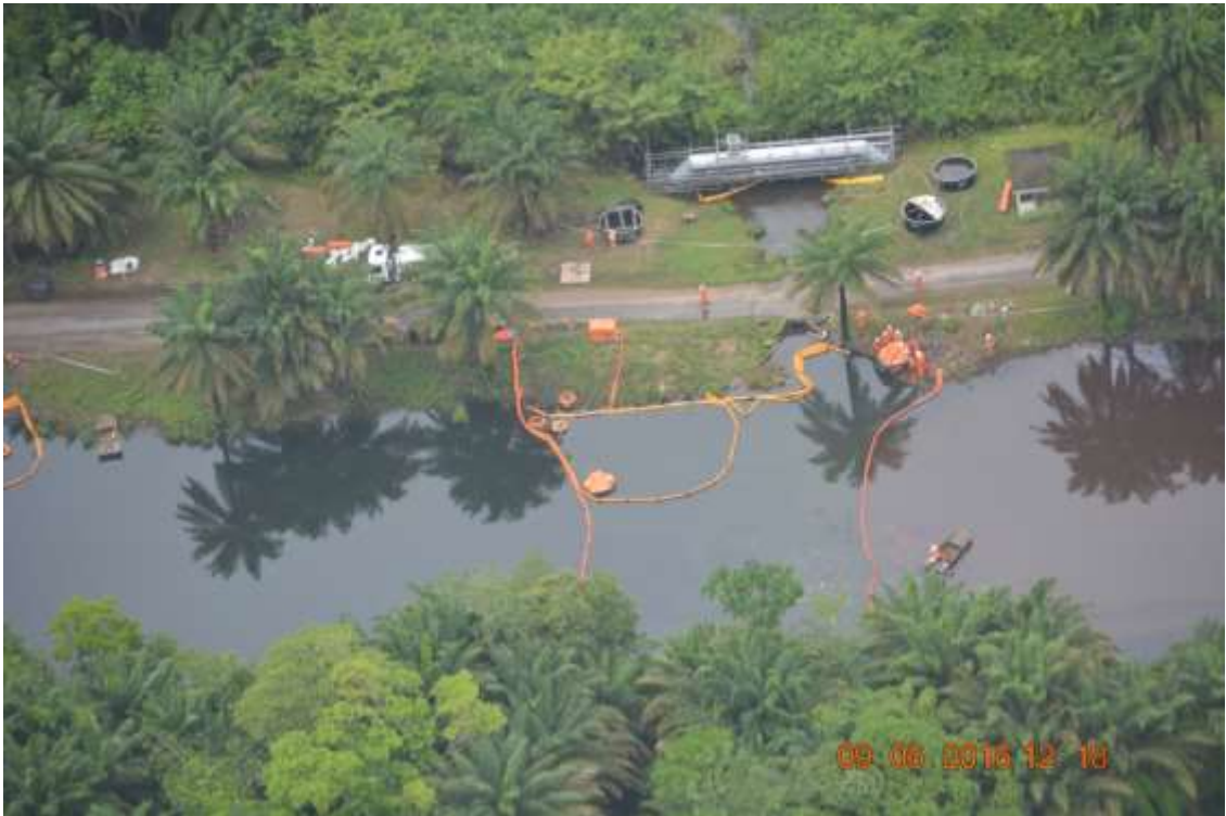
Overview: Part of spill impact on 48" Forcados Export Pipeline Right of Way at Ogulagha. Picture was taken during overfly on 9 th June 2016.
