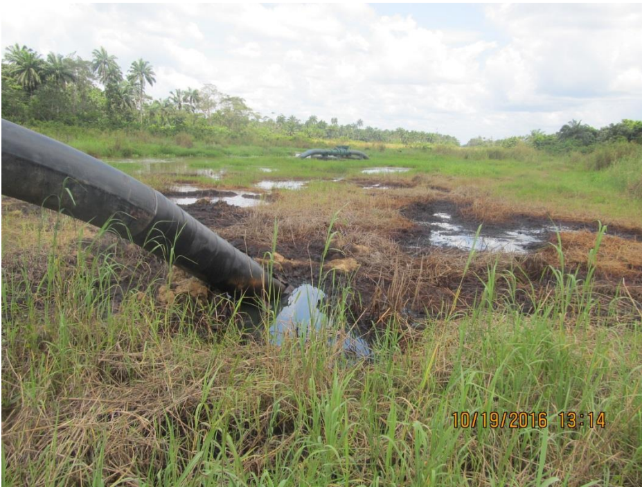
Overview: Part of spill impact on 20" Kolocreek-Rumuekpe Pipeline Riser at Aminigboko. Picture was taken during Joint Investigation of 19 th October 2016.
