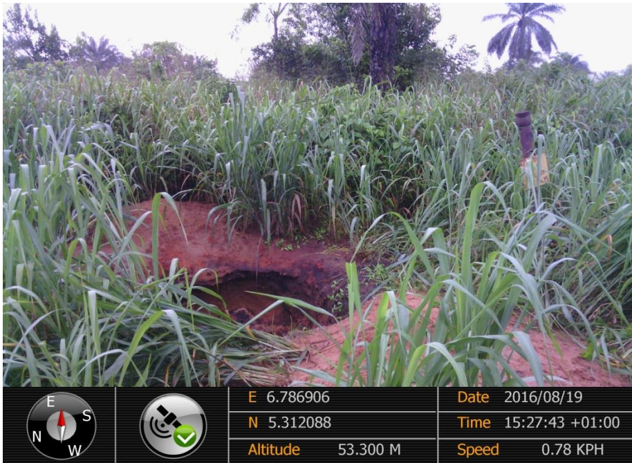
Overview: Part of spill impact on 18" Assa-Rumuekpe Pipeline at Ochia. Picture was taken during Joint Investigation of 19 th August 2016.
