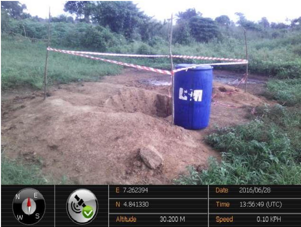
Overview: Part of spill impact on 8" Afam Well 27 T Flowline at Ayama. Picture was taken during Joint Investigation of 28 th June 2016.
