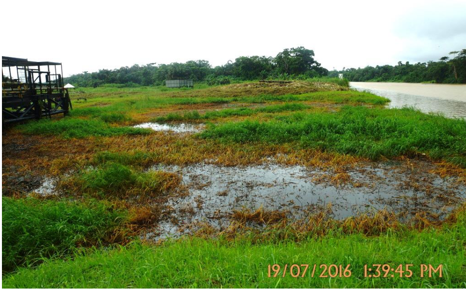
Overview: Part of spill impact on 16" Tunu-Brass Creek Pipeline Riser at Peretorugbene. Picture was taken during Joint Investigation of 19 th July 2016.
