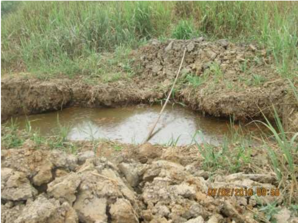
Overview: Part of spill impact on 16" Nun River – KoloCreek Pipeline Right of Way at Oporoma. Picture was taken during Joint Investigation of 7 th February 2016.
