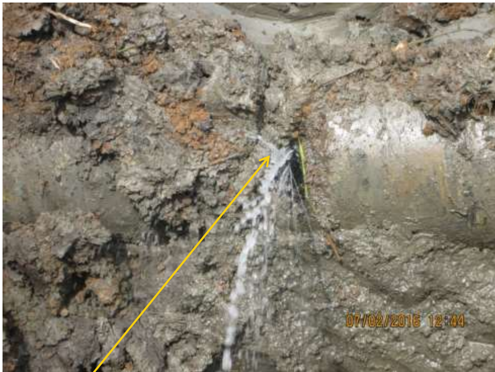
Close-up: Hacksaw cut on 16" Nun River – KoloCreek Pipeline at Oporoma. Picture was taken during Joint Investigation of 7 th February 2016.
