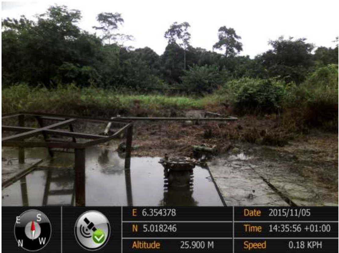
Overview: Spread of oil observed on Etelebou Well6T Right of Way. Picture was taken during Joint Investigation of 5 th November 2015.
