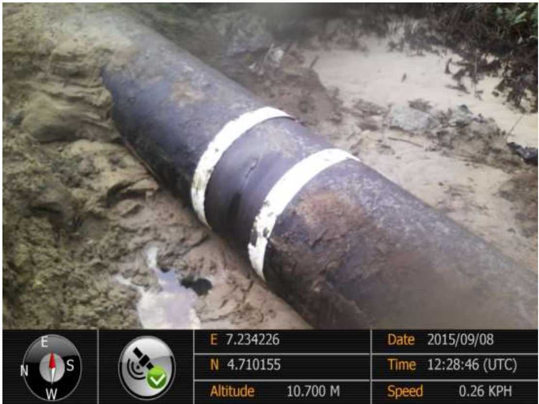
Overview: Part of spill impact on 28" Nkpoku-Bomu Pipeline Right of Way at Kporghor/Gio. Picture was taken during Joint Investigation of 8 th September 2015.
