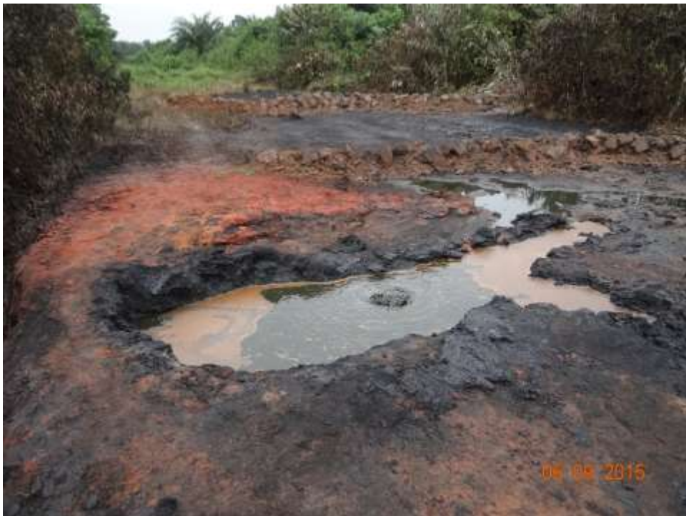
Overview: Part of spill impact on 28" Nkpoku-Bomu Pipeline Right of Way at Norkpo. Picture was taken during Joint Investigation of 6 th September 2015.
