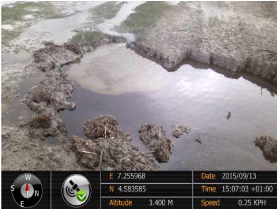
Overview: Part of spill impact on 28" Bomu-Bonny Pipeline Right of Way at Bodo West. Picture was taken during Joint Investigation of 13 th September 2015.
