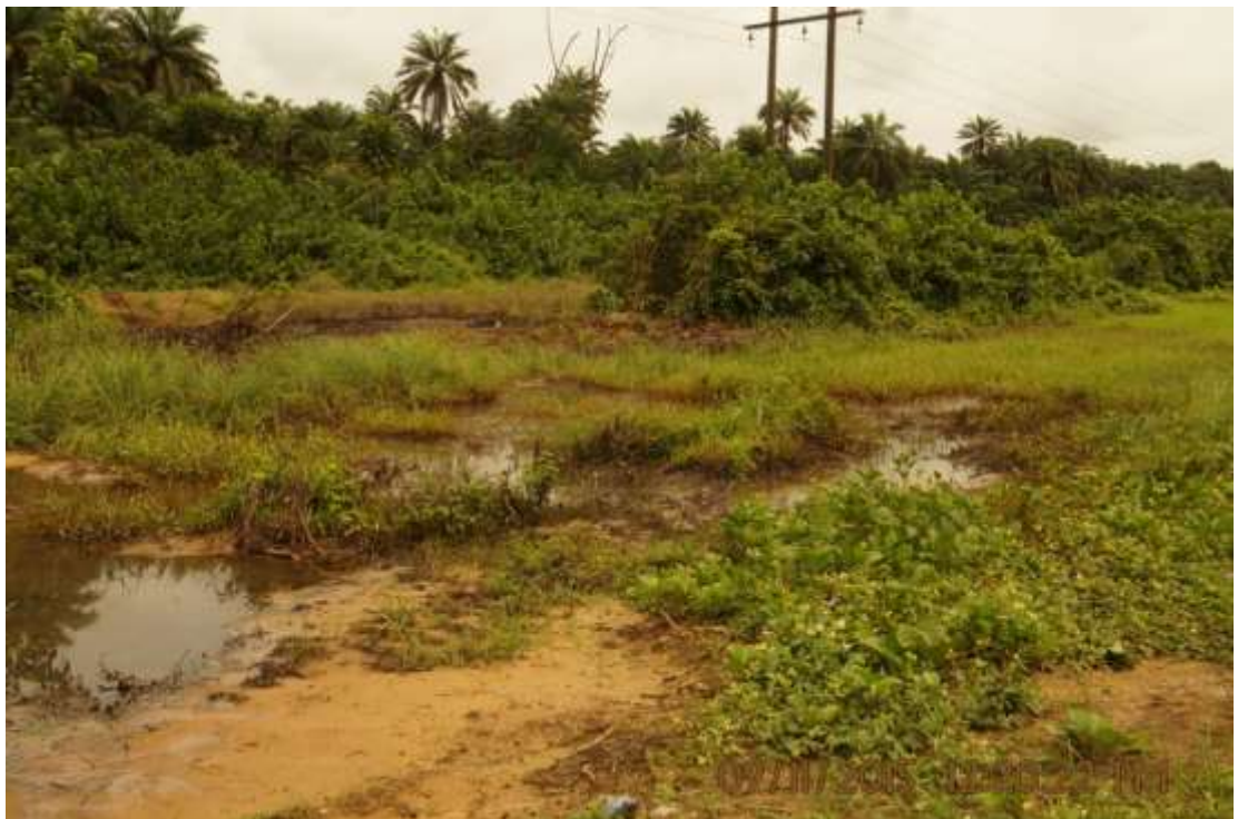
Overview: Part of spill impact on 24" Trans Escravos Pipeline Right of Way at Obotobo. Picture was taken during Joint Investigation of 9 th November 2015.
