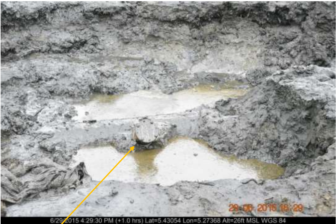
Close-up: Illegal fitting on 24" Trans-Escravos Pipeline at Sokebolou. Picture was taken during Joint Investigation of 29 th June 2015.
