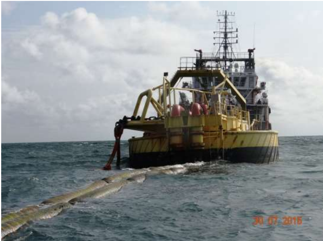
Overview: No visible impact on Bonny Terminal Single Point Mooring (SPM) 1 at Bonny. Picture was taken during Joint Investigation of 30 th July 2015.
