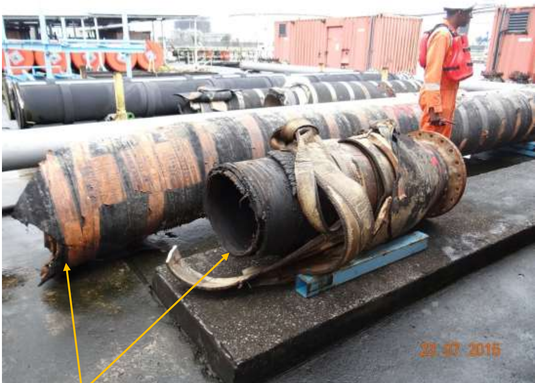
Close-up: Complete Rupture of Floating Hose 13 on Bonny Terminal Single Point Mooring (SPM) 1 at Bonny. Picture was taken during Joint Investigation of 23 rd July 2015.
