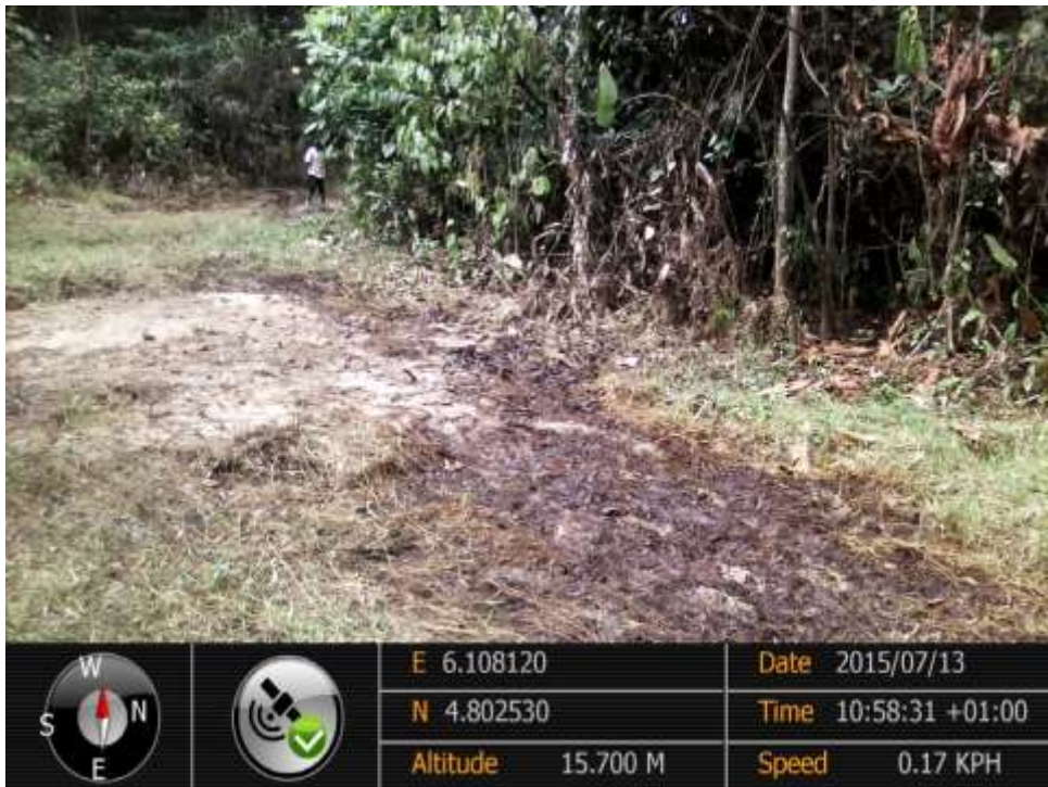
Overview: Part of spill impact on 10" Diebu Creek – Nun River Pipeline Right of Way at Oporoma. Picture was taken during Joint Investigation of 13 th July 2015.
