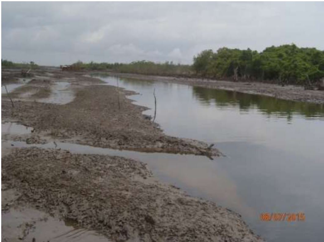
Overview: Part of spill impact on 28" Bomu-Bonny Pipeline Right of Way at Owokiri. Picture was taken during Joint Investigation of 8 th July 2015.
