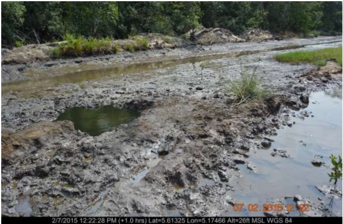
Overview: Part of spill impact on 20" Otumara-Escravos Pipeline Right of Way at Ugboegungun. Picture was taken during Joint Investigation of 7 th February 2015.
