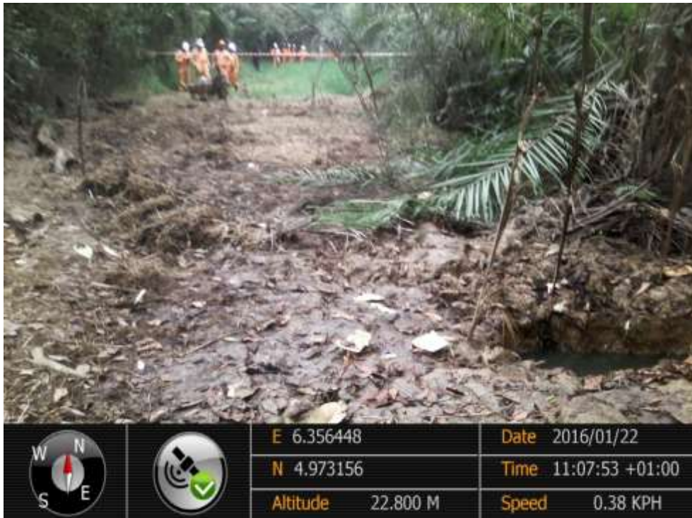
Overview: Part of spill impact on 8" Etelebou – KoloCreek Pipeline Right of Way at Etegwe/Okutukutu. Picture was taken during Joint Investigation of 22 nd January 2016.
