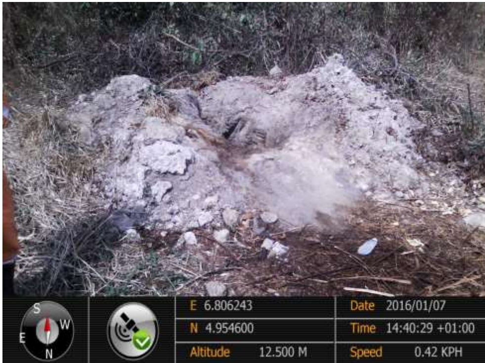
Overview: Part of spill impact on 20" Rumuekpe – Nkpoku Pipeline Right of Way at Omukpobu-Ibaa. Picture was taken during Joint Investigation of 7 th January 2016.
