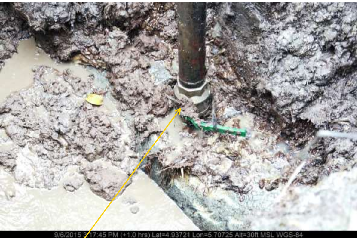
Close-up: Illegal fitting on 20" Opukushi-BrassCreek Pipeline at Tamogbene. Picture was taken during Joint Investigation of 6 th September 2015.
