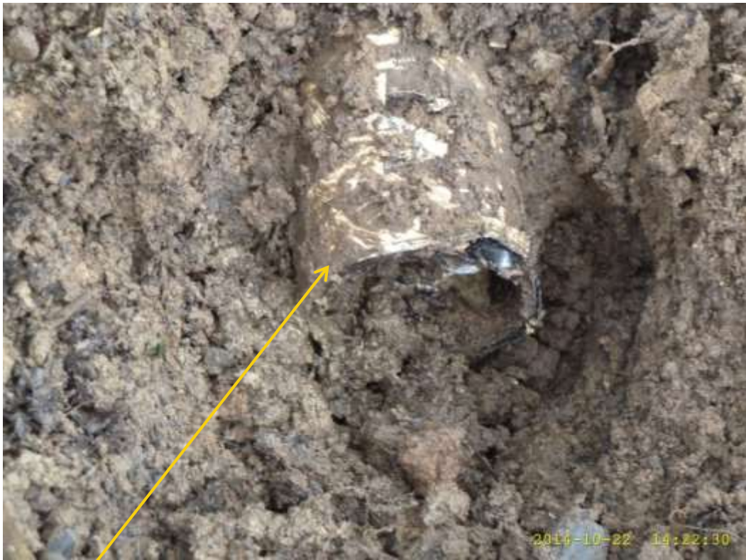
Close-up: Cut section of 4" KoloCreek Well3T Flowline at Otusega. Picture was taken during Joint Investigation of 22 nd October 2014.
