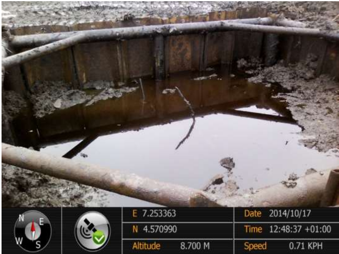
Overview: Part of spill impact within cofferdam on 28" Bomu-Bonny Pipeline Right of Way at Bodo City. Picture was taken during Joint Investigation of 17 th October 2014.
